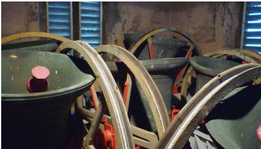
The bells after the refurbishment
